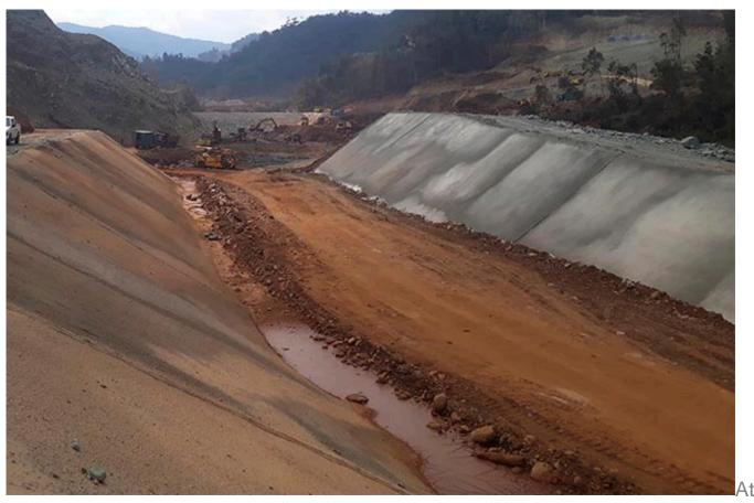
6:55 a.m. this Sunday morning, the workers of the Engineering Works Construction Company No. 16 completed the lining of the diversion channel in the construction of the Levisa Dam, which closes the first stage in the execution of this work.
